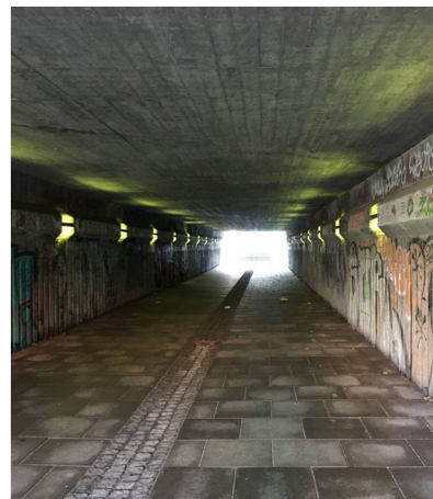
Tunnel under Randersvej
